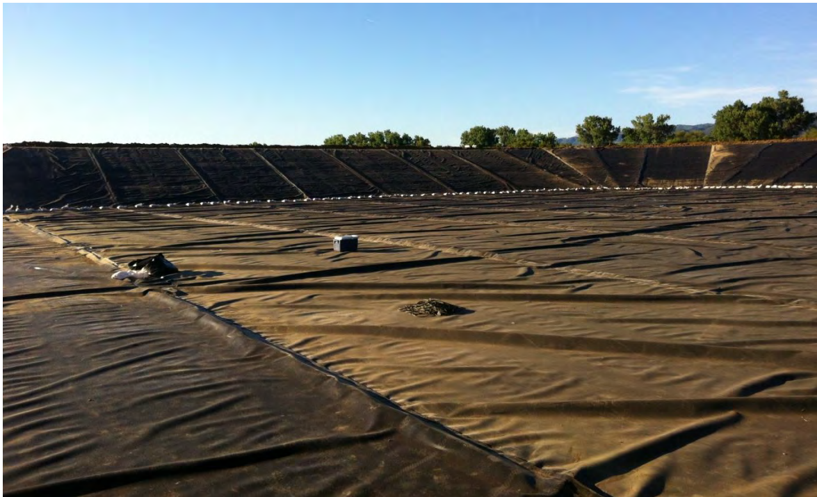
Figure 164. Installation of liner on offstream pond
