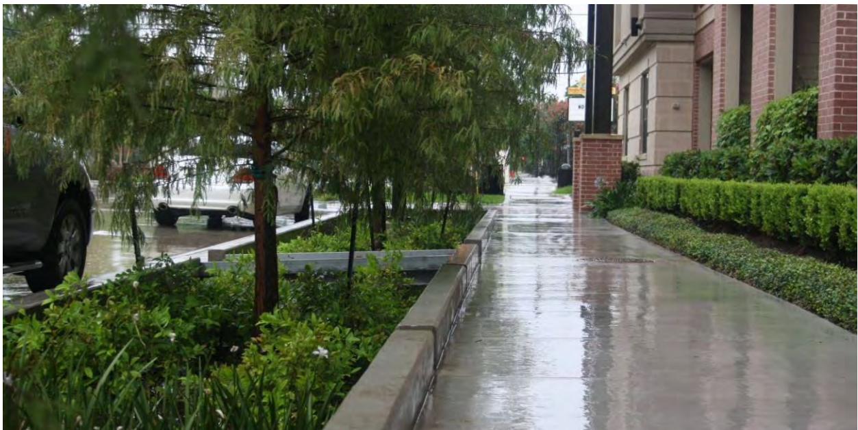
Figure 182. Bioretention facilities in downtown areas
