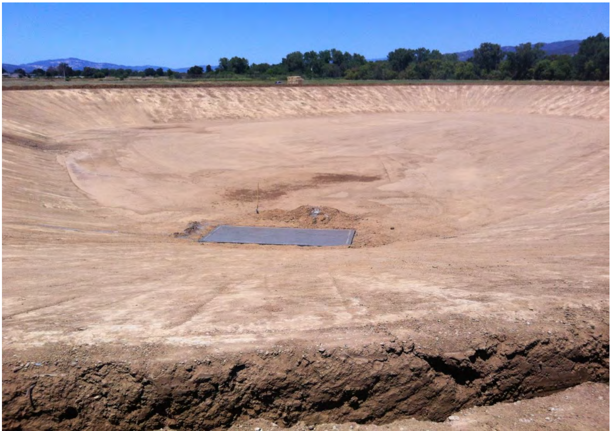
Figure 163. Offstream pond before and during grading
