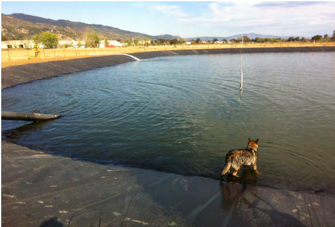
Figure 165. Offstream pond partially filled with freshwater
