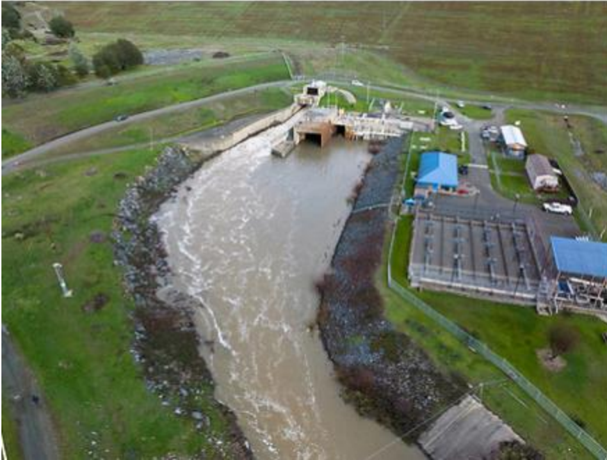
January 14, 2023, Coyote Valley Dam. Photo by Kenneth James, DWR
