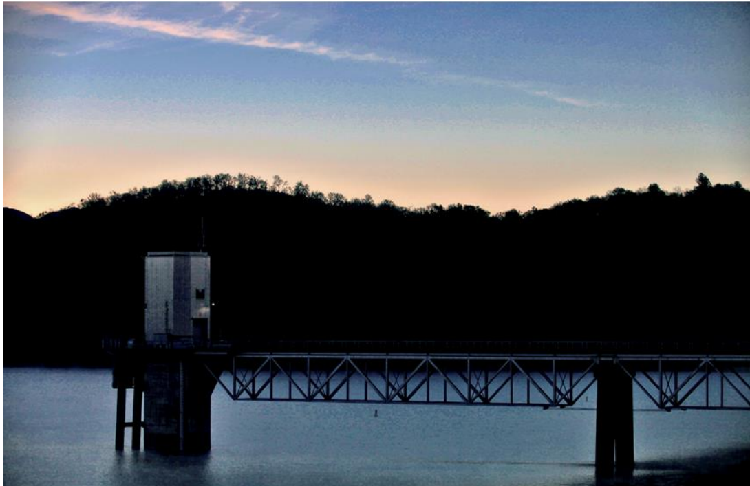
At Coyote Valley Dam, Lake Mendocino. Photo by CJ Watt, 1/22/23
