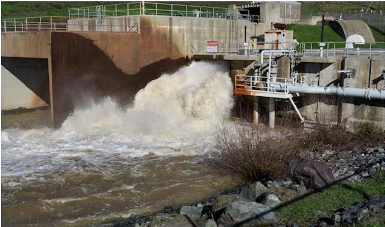
January 16, 2023, Coyote Valley Dam flood release Photo by Karen Rifkin
