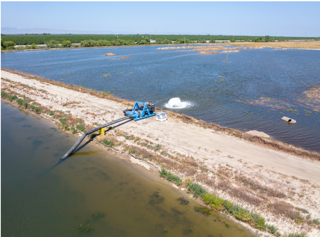
A drone view of the James Irrigation District utilizing pumps from DWR’s Emergency Pump Program in May 2023 to divert water and fill a basin for groundwater recharge in Fresno County. DWR supplied temporary pumps and equipment along the Kings and the Kaweah rivers in the Tulare Lake basin to divert floodwater off these rivers and reduce flood impacts in the former Tulare Lake lakebed. Local agencies were able to divert an estimated 20,517 acre-feet of floodwater for recharge in the Tulare Lake region from late April to late June.
