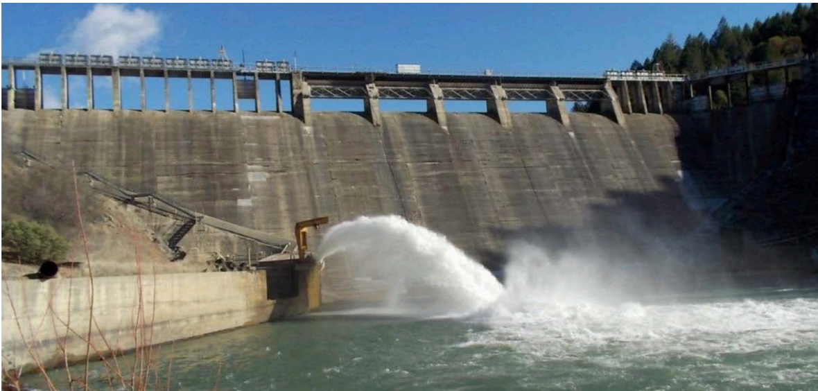
Scott Dam Spillway
